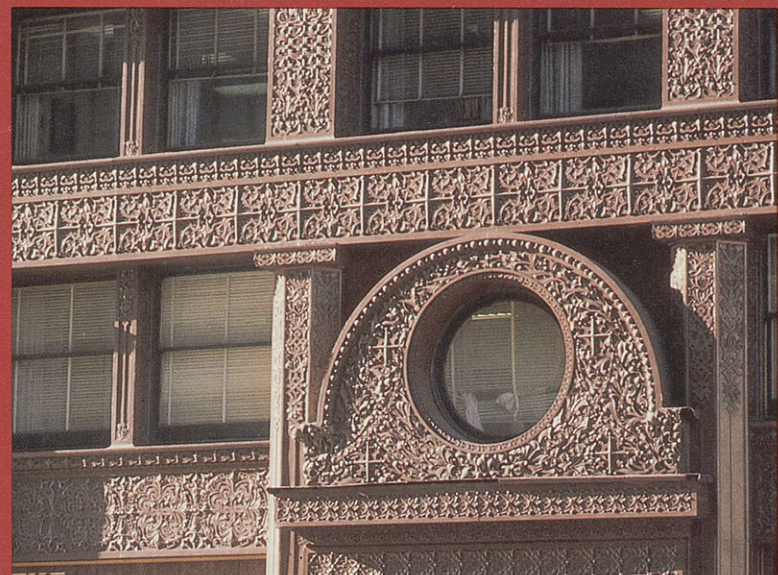
Detail of the entrance to the Rockefeller Building
