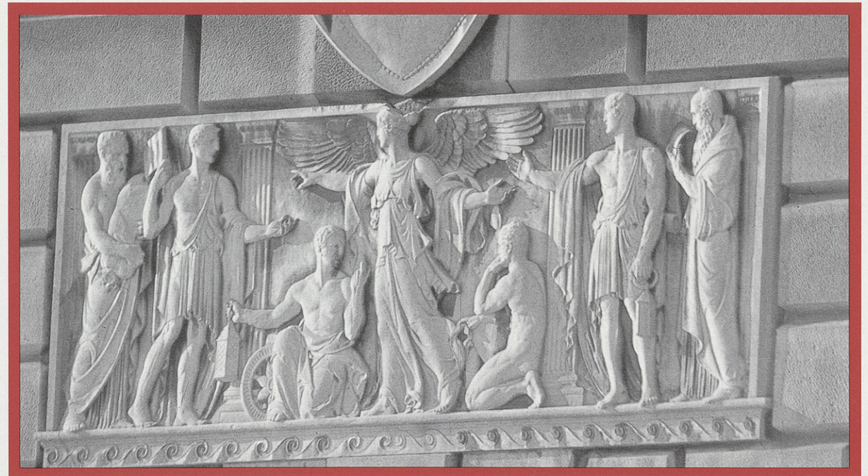
Detail of Brotherhood of Railway Trainmen Building
