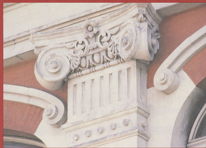
Detail of restored plaster work in the State Theater
