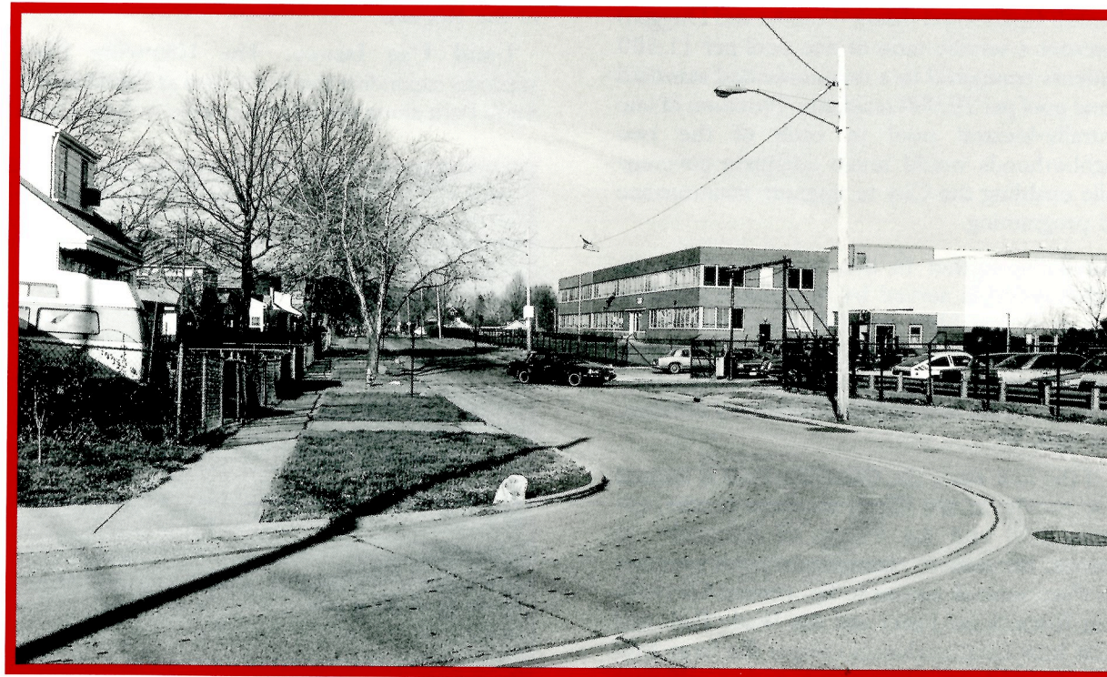
Poorly-designed parking lot access results in excessive through-traffic on residential streets adjacent to industrial facilities. (LOCATION: East 185th Street, south of St. Clair Avenue).
