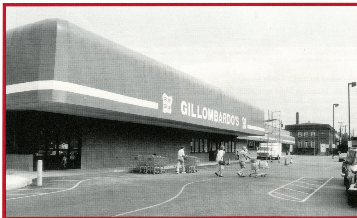
Construction of a new shopping plaza demonstrates the continued viability of retailing in the Broadway neighborhood. (LOCATION: Broadway and Cable).
