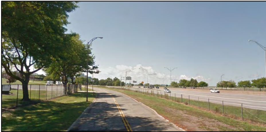
South Marginal Road looking west at East 40 th Street
